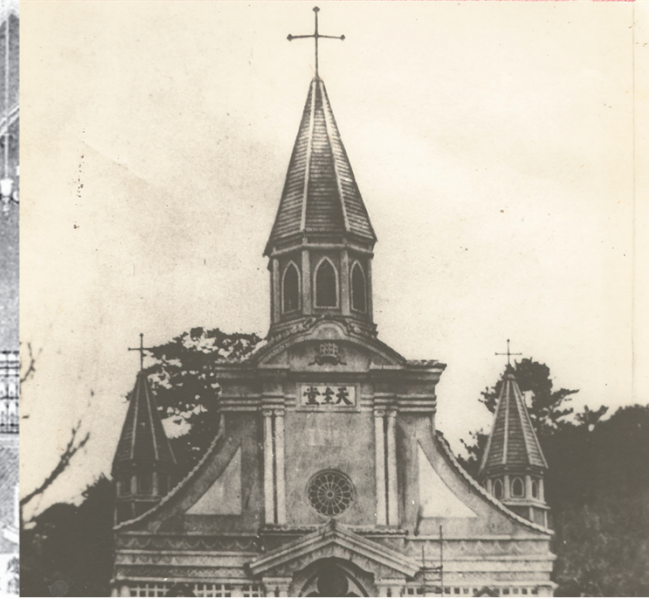
Oura Cathedral (component ⑫) at the time of its construction * Photo reprinted by courtesy of Nagasaki Bunkensha
